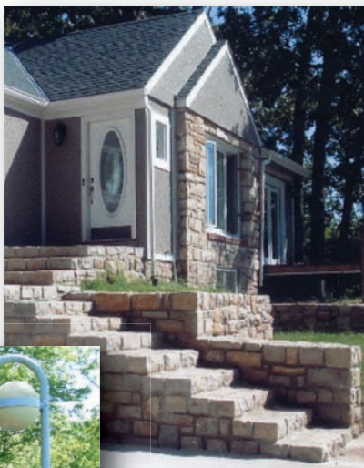
Retaining Walls Steps
